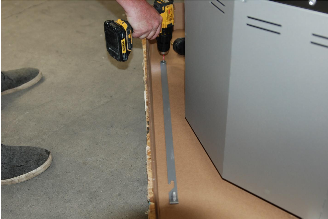
Figure 6 – Remove Lid Prop Bar
