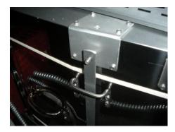
Place the lid support bar onto the stud as shown.
